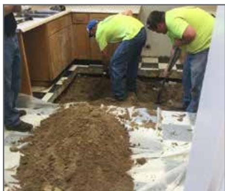
ABOVE: K1 in the midst of the pipe construction, September 2016.
